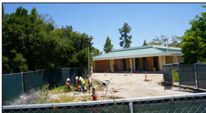
ONGOING CAMPUS CONSTRUCTION. PHOTO BY LOGAN MURPHY.
